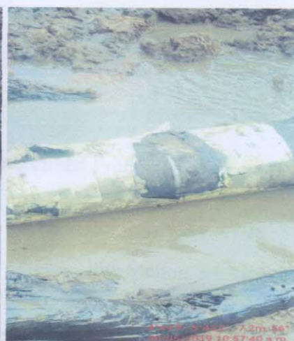
FIG H: Incident point after repairs
